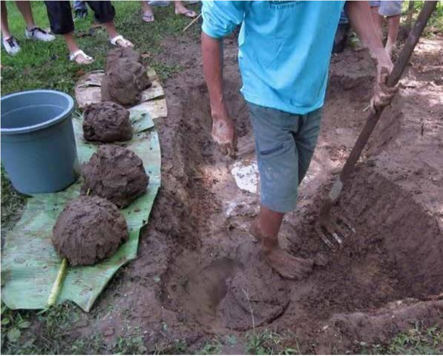
Pic 5. Flatten the mixture of applied soil Source : facebook green architecture, 2011
