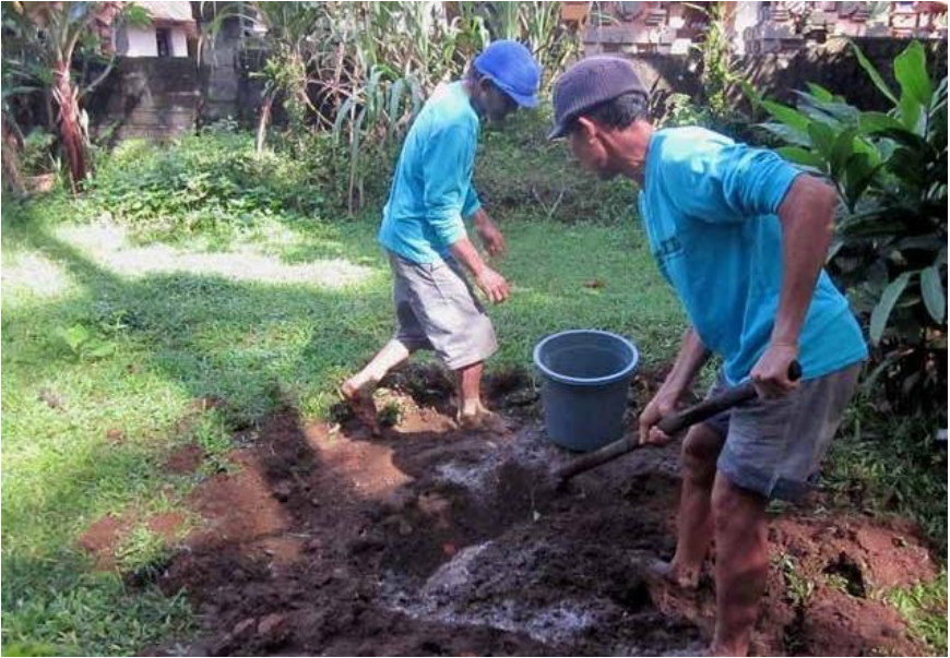
Pic 2. Process of mixing soil with water Source: facebook green architecture, 2011
